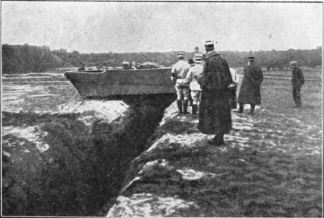
FIG. 9. — TRACTEUR HOLT ALLONGÉ TRAVERSANT UNE TRANCHÉE DE DEUX MÈTRES
